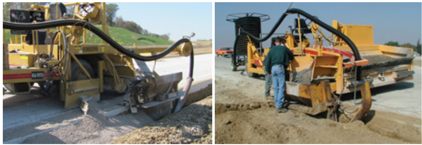
Figure 7.13. Automated equipment installing CPE edgedrains (courtesy of Kevin Merryman, Iowa DOT)
