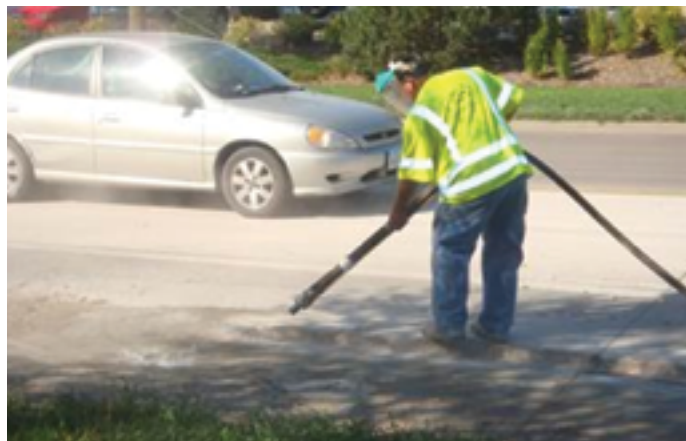
Figure 5.17. Sandblasting to remove loose debris
