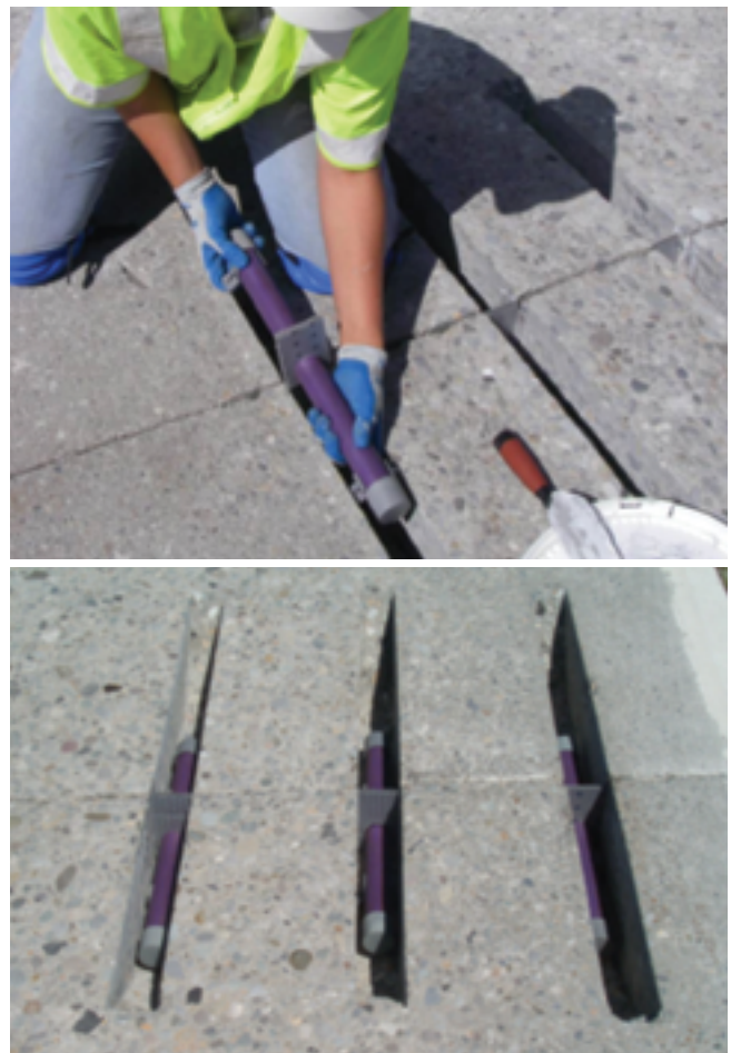
Figure 8.14. Placing dowel bar assembly into the slot (Pierce, Uhlmeier, and Weston 2009)
