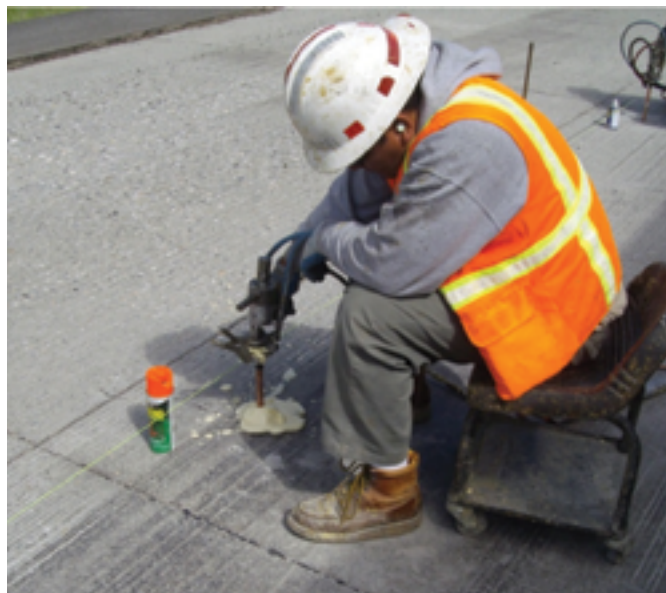
Figure 4.10. Injecting polyurethane (photo courtesy of WSDOT)
