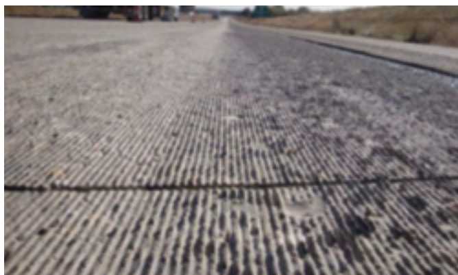
c. Conventional diamond ground surface
