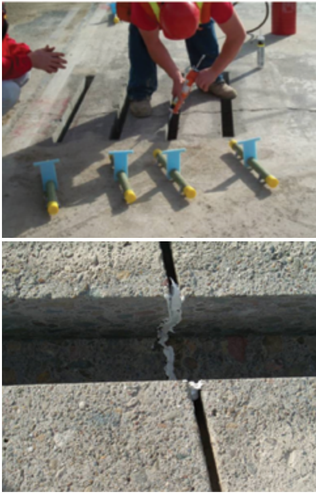
Figure 8.13. Applying caulk on slot sides and bottom (Pierce, Uhlmeier, and Weston 2009)
