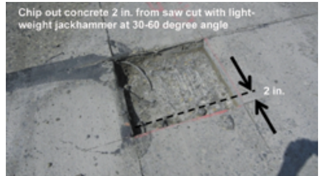
Figure 5.11. Repair area prepared using the saw-and-patch (Type 1) procedure (Frentress and Harrington 2012)
