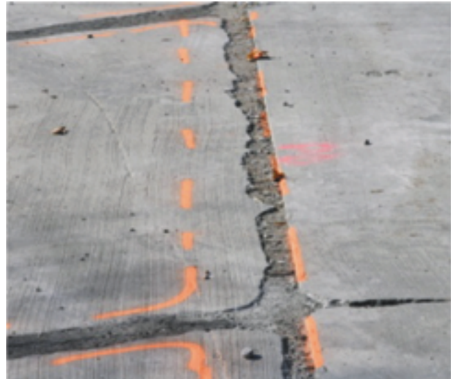
Figure 5.10. Repair boundaries marked for sawing (Frentress and Harrington 2012)
