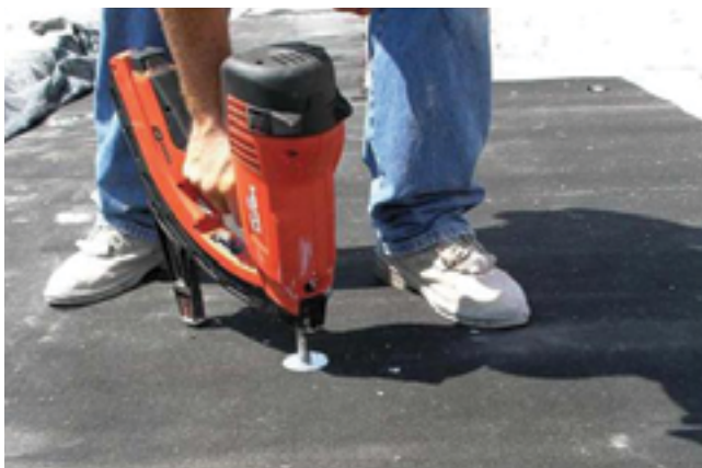
Figure 11.18. Fastening nonwoven geotextile interlayer (Harrington and Fick 2014)
