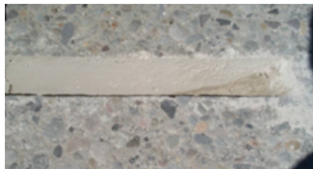
a. Debris and saw blade slurry on side of slot
