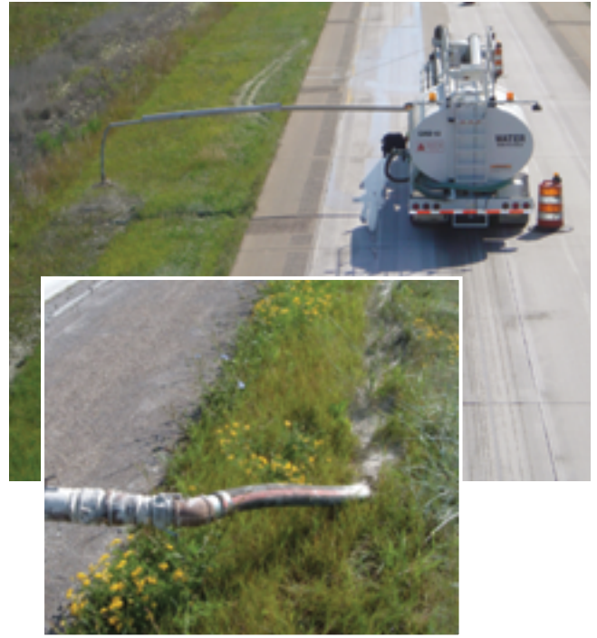
Figure 9.19. Depositing slurry on vegetated slopes in rural areas (IGGA 2010)
