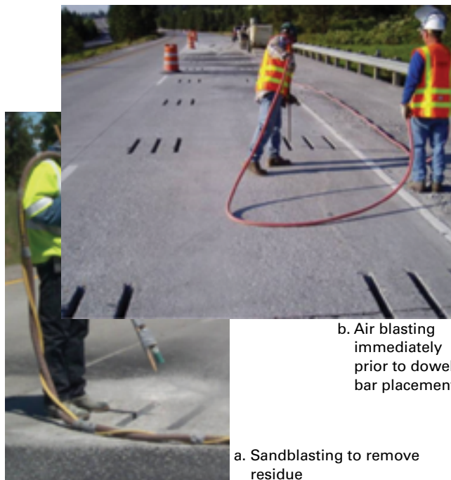
Figure 8.11. Preparing dowel bar slot (Pierce, Uhlmeyer, and Weston 2009)
