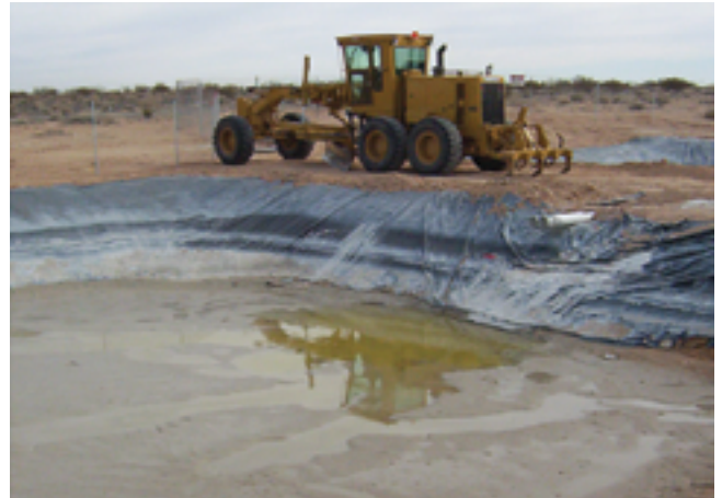
Figure 9.20. Vacuum system (top) and slurry deposit in settlement pond (bottom) (IGGA 2010)
