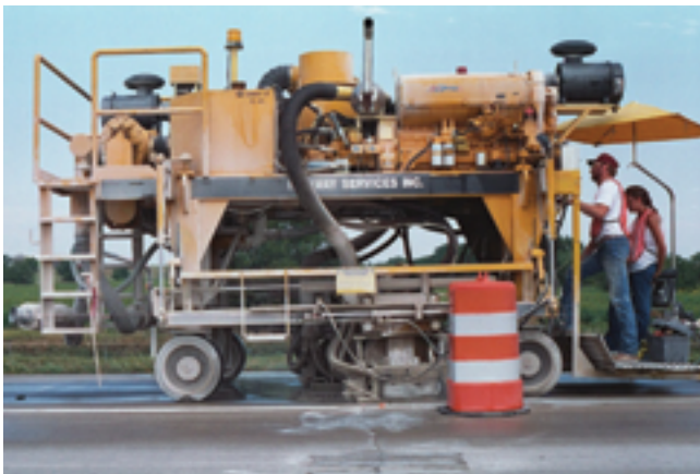
Figure 8.6. Example of diamond-bladed slot-cutting machine (Pierce, Uhlmeyer, and Weston 2009)
