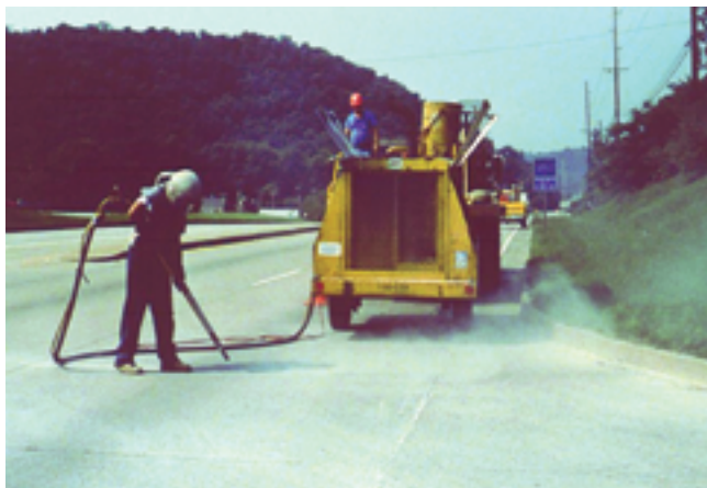
Figure 10.9. Sandblasting along a transverse joint
