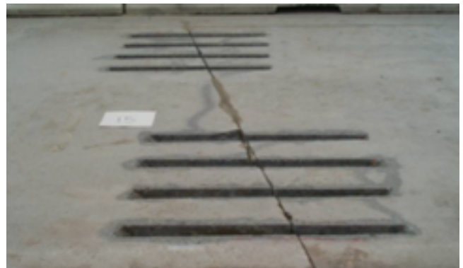
b. Skewed transverse joints
