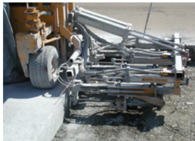
Figure 6.12. Example of gang drill used for dowel bar installation
