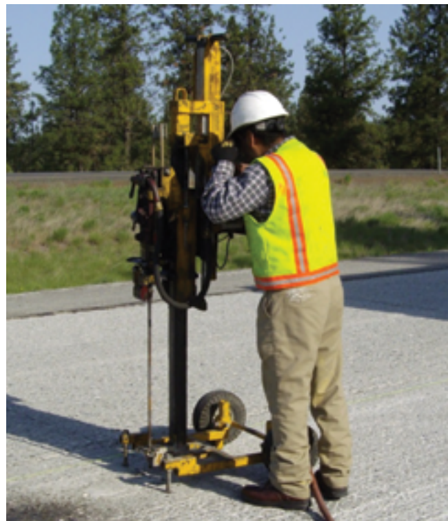
Figure 4.8. Drilling injection holes (photo courtesy of WSDOT)
