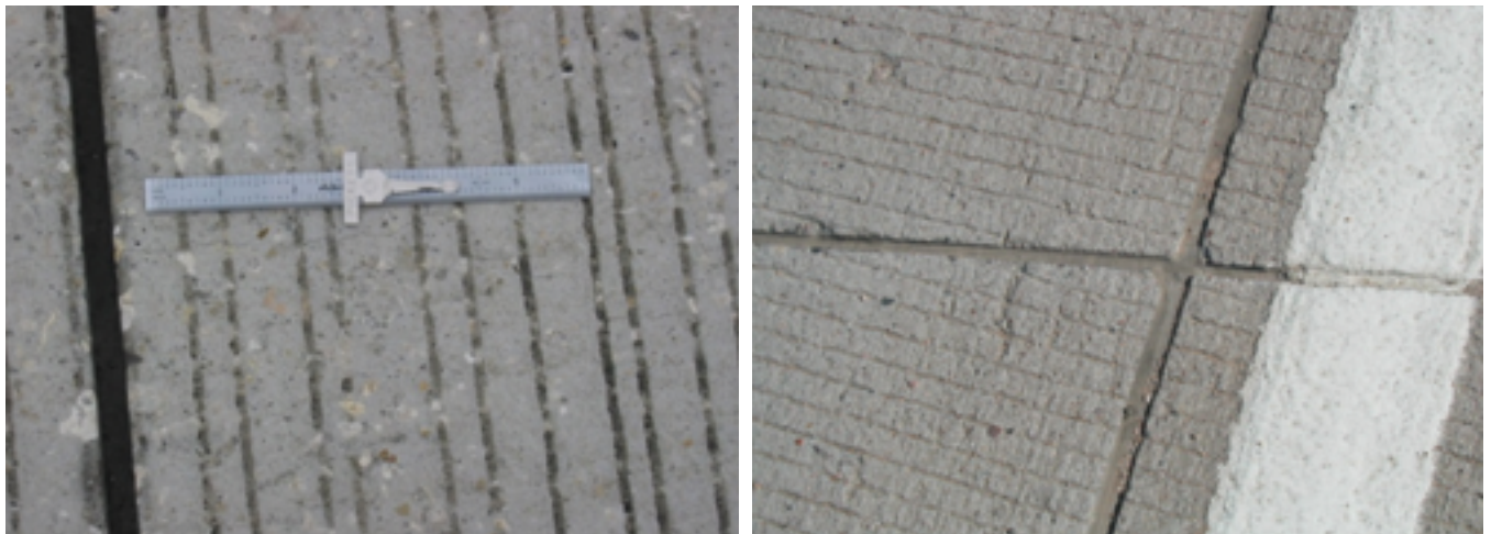
Figure 10.2. Hot-applied thermoplastic (left) and silicone (right) sealants
