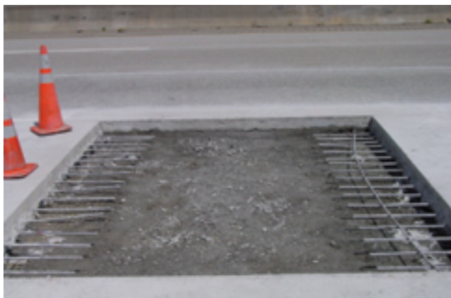
Figure 6.11. Prepared CRCP repair area with exposed reinforcing steel (Gulden 2013).
