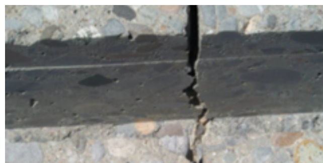
b. Final cleaned slot surface
