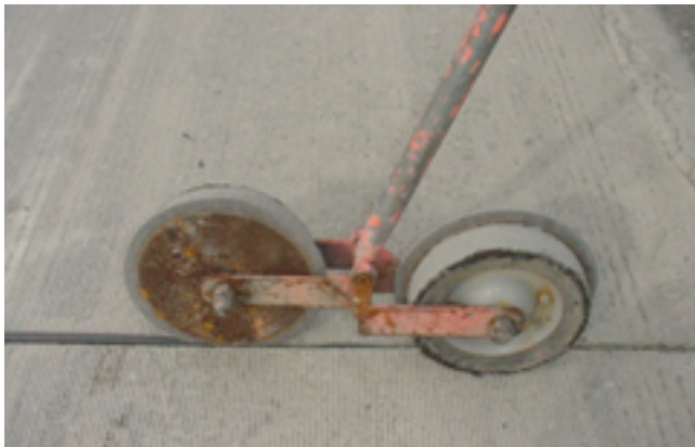
Figure 10.10. Installation of the backer rod
