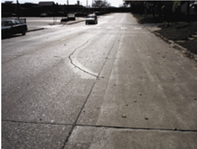
Figure 5.25. Diamond grinding of PDR (Frentress and Harrington 2012)
