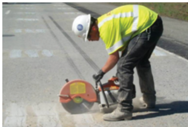
Figure 8.17. Re-establishing the transverse joint in patching material (Pierce, Uhlmeier, and Weston 2009)
