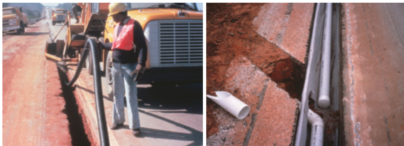
Figure 7.7. Corrugated (left) and rigid (right) pipe edgedrains
