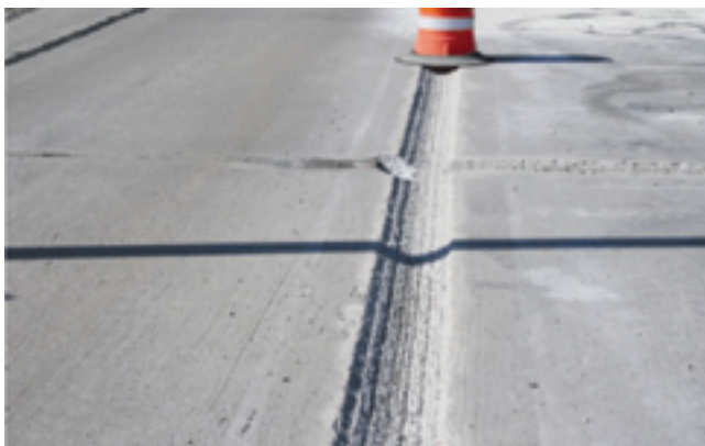
Figure 5.15. Rock saw capable of producing rounded milling (top) and milling pattern (bottom) (Frentress and Harrington 2012)
