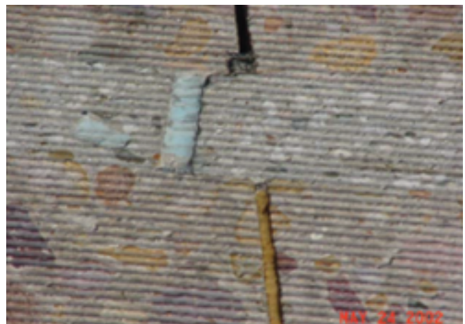
d. Misaligned foam core board
