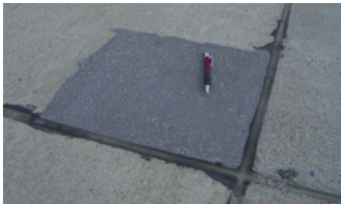
Figure 5.19. Partial-depth repair featuring a proprietary polymer-based repair material
