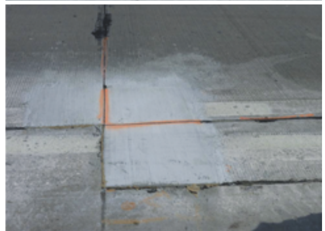
Figure 5.23. Completed joint repairs (Frentress and Harrington 2012)
