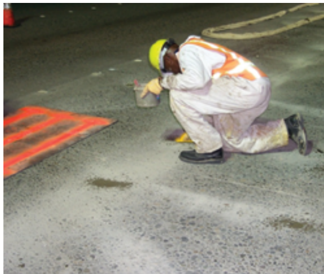
Figure 4.9. Patching drill holes (photo courtesy of WSDOT)
