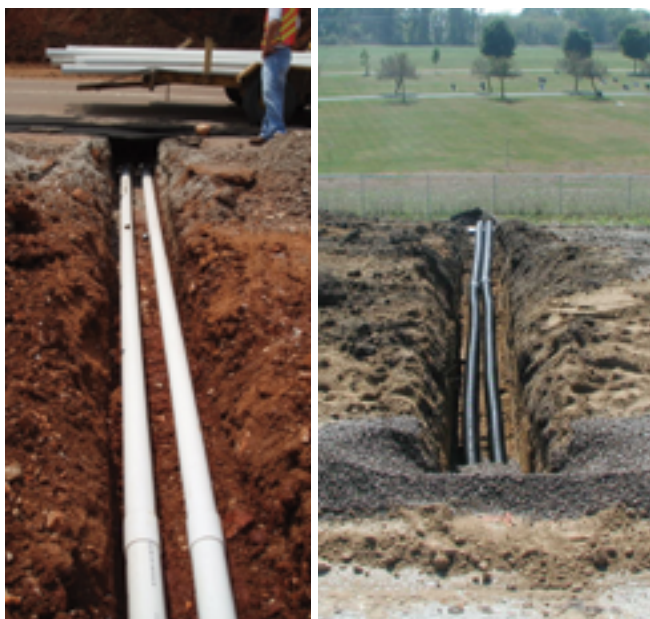
Figure 7.14. Lateral outlet pipes (courtesy of John Donahue [left] and Kevin Merryman [right])
