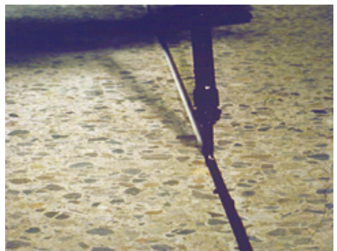
Figure 10.11. Installation of hot-applied joint sealant
