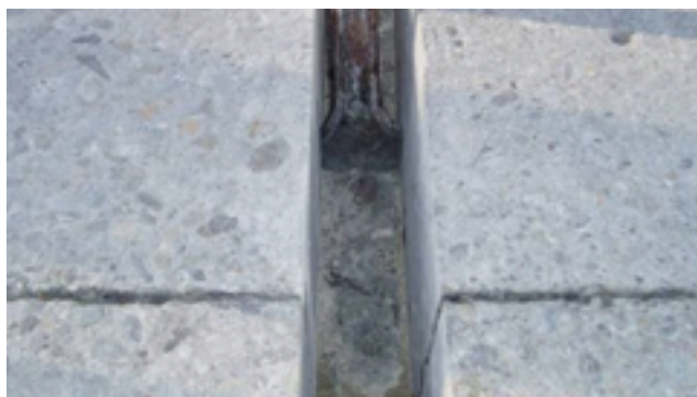
Figure 8.10. Leveling the bottom of the dowel bar slot (Pierce, Uhlmeyer, and Weston 2009)
