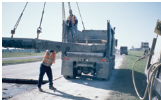
Figure 6.10. Lift-out method of slab removal
