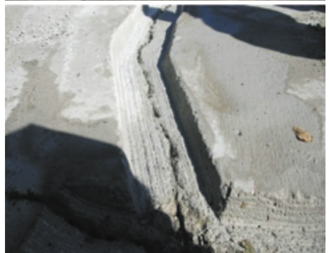
Figure 5.16. Vertical edge mill head (top) and milling pattern (bottom) produced by the vertical edge mill head (Frentress and Harrington 2012)
