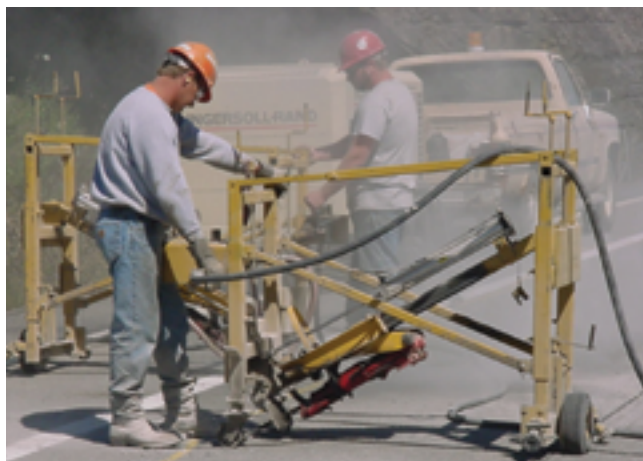
Figure 8.19. Drilling holes for cross stitching
