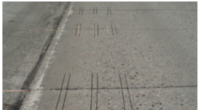
a. Nonskewed transverse joints
