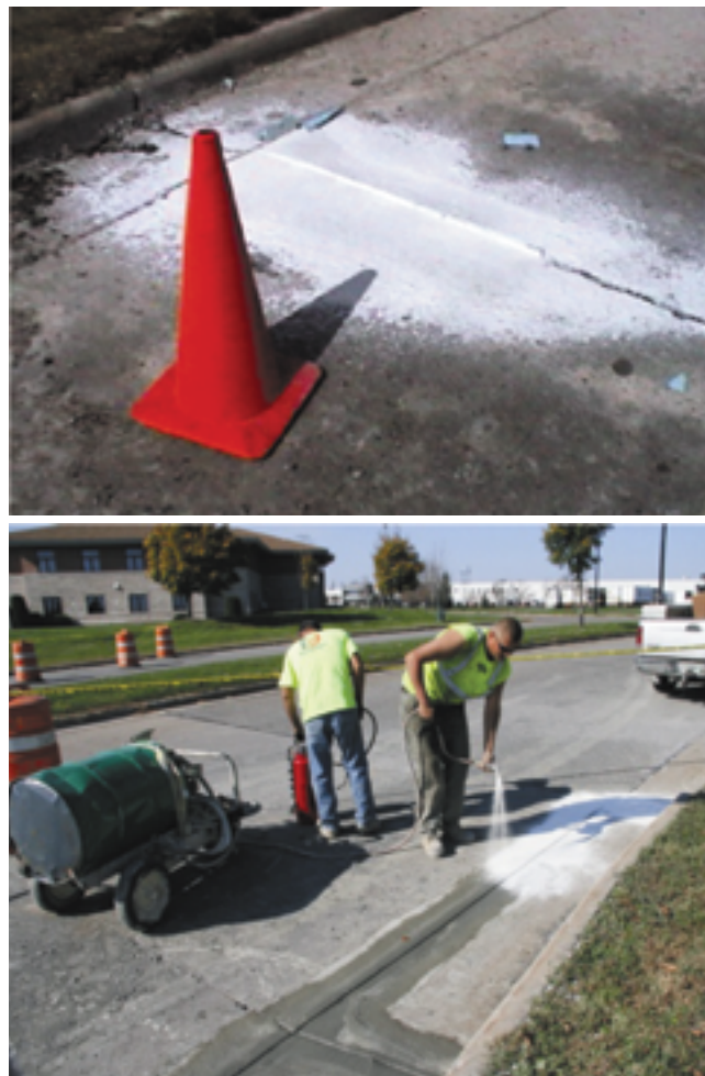
Figure 5.24. Repair material curing operation (Frentress and Harrington 2012)
