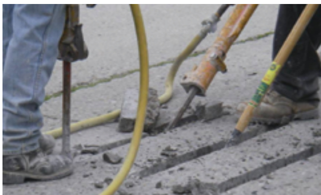
Figure 8.9. Operating jackhammers at no more than a 45-degree angle (Pierce, Uhlmeyer, and Weston 2009)
