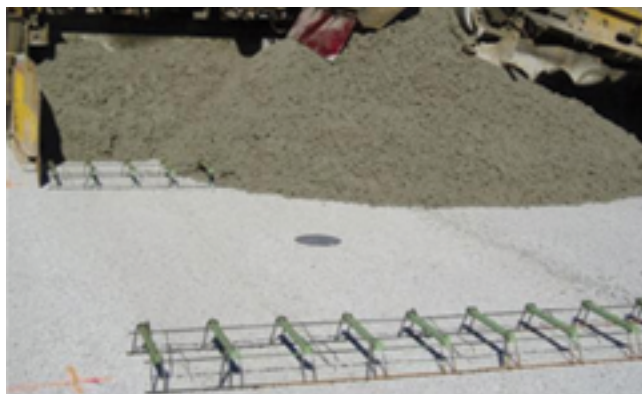
Figure 3.16. Placement of metal reflector prior to paving (Ye and Tayabji 2009)
