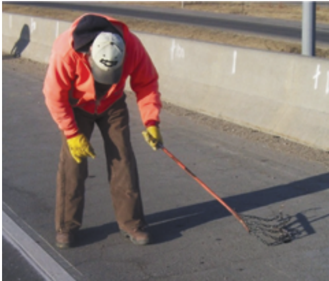
Figure 5.9. Sounding deteriorated concrete using hammer (top) and chain (bottom) (Frentress and Harrington 2012)
