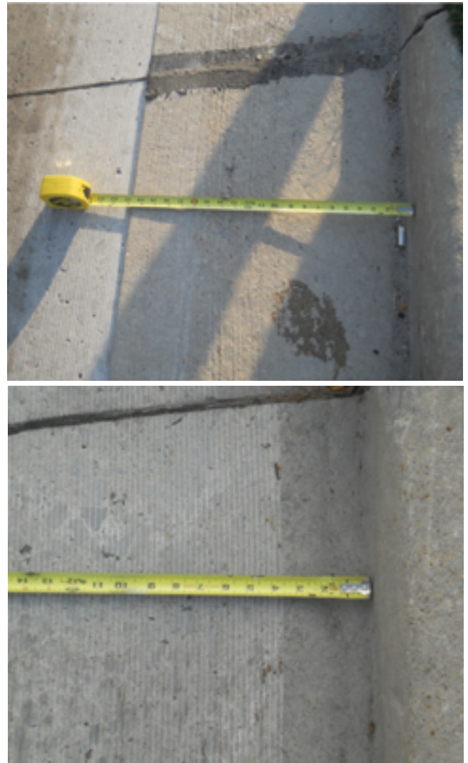
Figure 9.17. Gutter apron before (top) and after (bottom) feathering pass (courtesy of Dan Frentress, IGGA)
