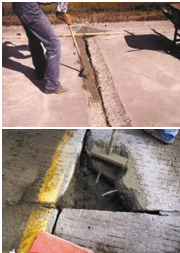
Figure 5.20. Application of cement grout as bonding agent (Frentress and Harrington 2012)
