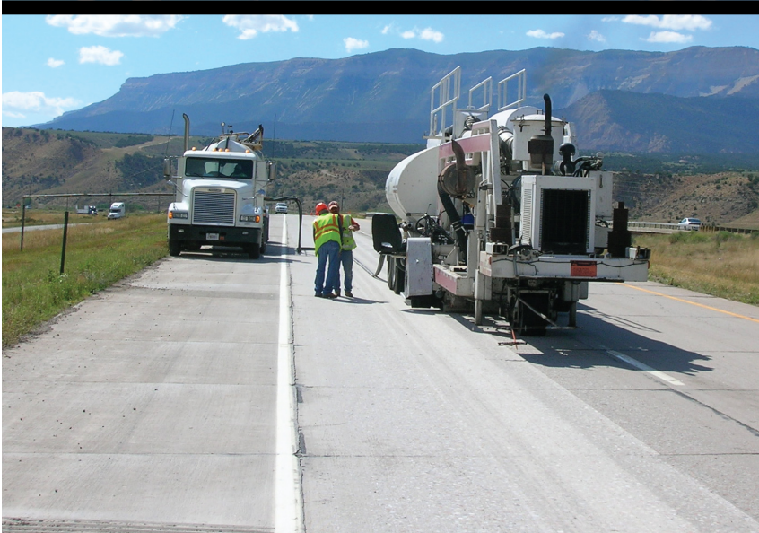
<< Diamond Grinding of I-70 in Colorado
