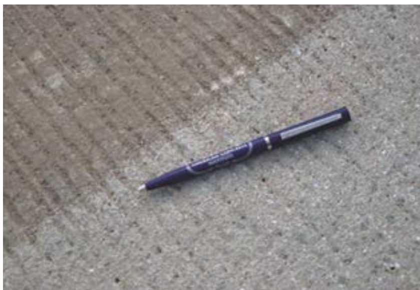
Figure 109. Compare the surface texture of the nonshotblasted area (upper left half of image) to the roughened surface texture on the shotblasted section of pavement (under the pen) (source: Leif Wathne, ACPA)
