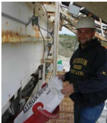
Figure 124. Fibers added at plant (left) and bags tossed into ready-mix truck (right) (source: Randell Riley, Illinois chapter, ACPA)
