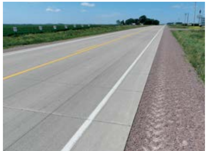
Figure 35. Poor to deteriorated asphalt pavement resurfaced with unbonded concrete overlay (source: Kevin Merryman, Iowa DOT)
