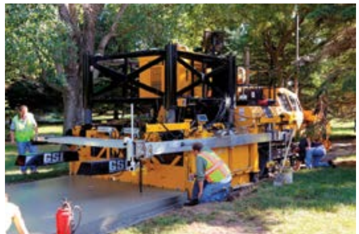
Figure 101. Zero clearance stringless paver (source: GOMACO)
