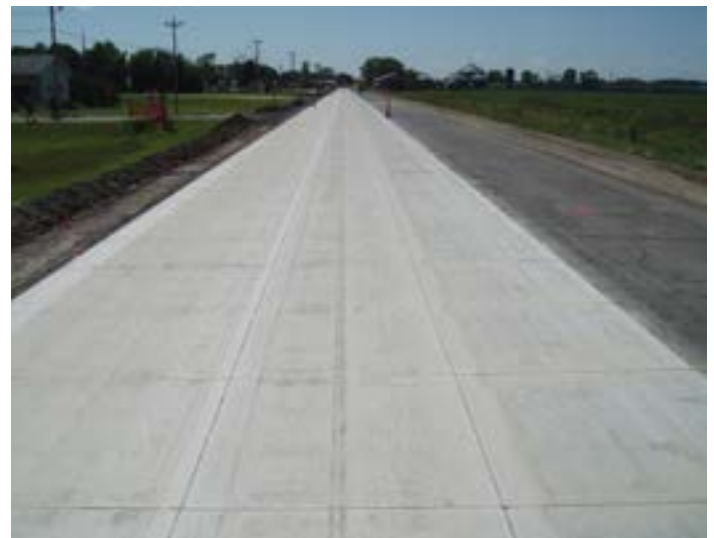
Figure 25. Bonded on composite pavement (source: James Cable, Iowa State University)
