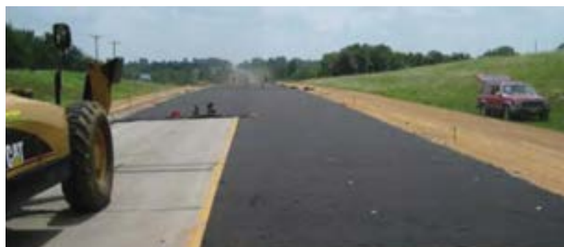
Figure 50. Geotextile fabric separation layer (source: Missouri DOT)
