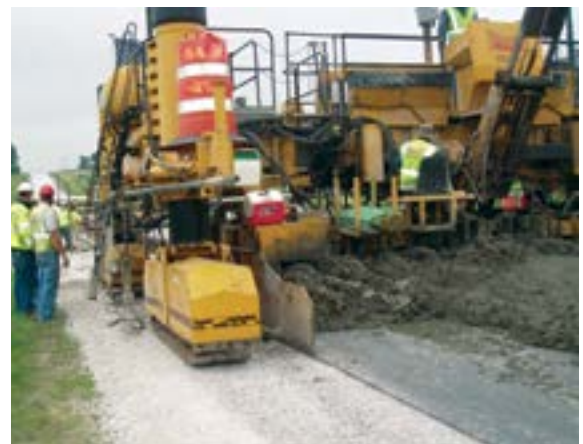
Figure 100. Stringless paver (source: Jim Cable, Iowa State University)
