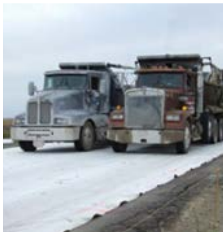
Figure 113. Paving on top of white geotextile fabric interlayer (source: Larry Engbrecht, South Dakota chapter, ACPA)
