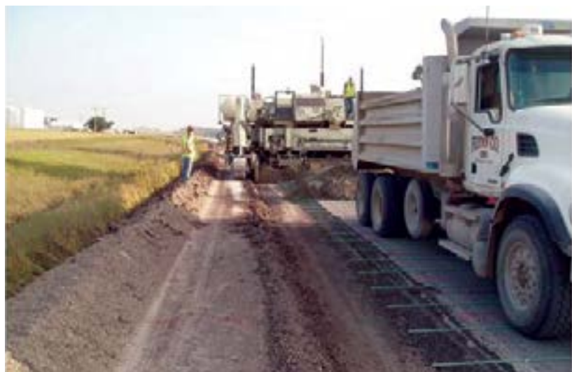
Figure 82. View of tiebars for concrete overlay widening unit
