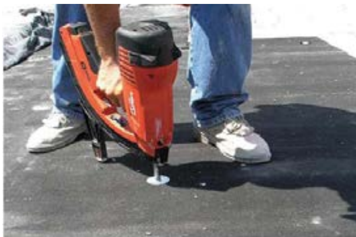
Figure 111. Fastening nonwoven geotextile fabric to existing concrete pavement
