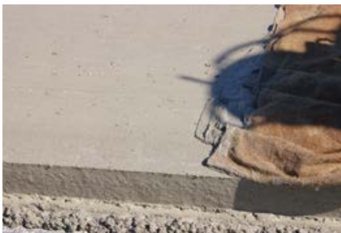
Figure 125. Finished concrete overlay with synthetic fibers
