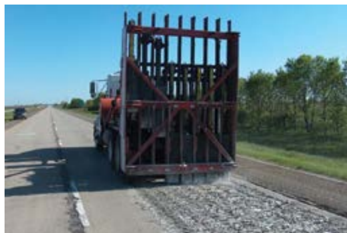
Figure 122. Rubblized concrete pavement (source: Todd Hanson, Iowa DOT)
