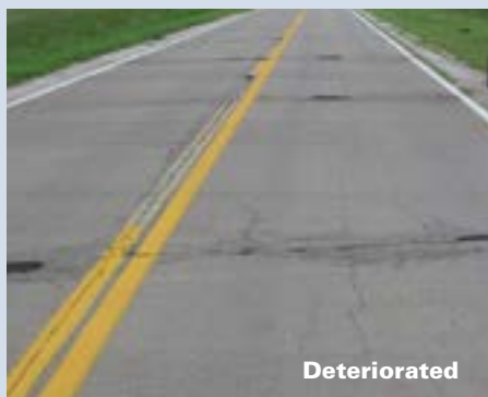
Figure 7. Pavement evaluation process, with examples of existing pavement conditions (source: Snyder & Associates, Inc.)
