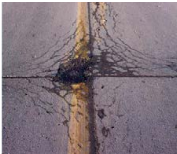
Figure 11. D-cracked pavement
