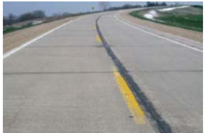
Figure 29. Three-inch concrete bonded overlay (photo dated 2013) (source: Todd Hanson, Iowa DOT)
