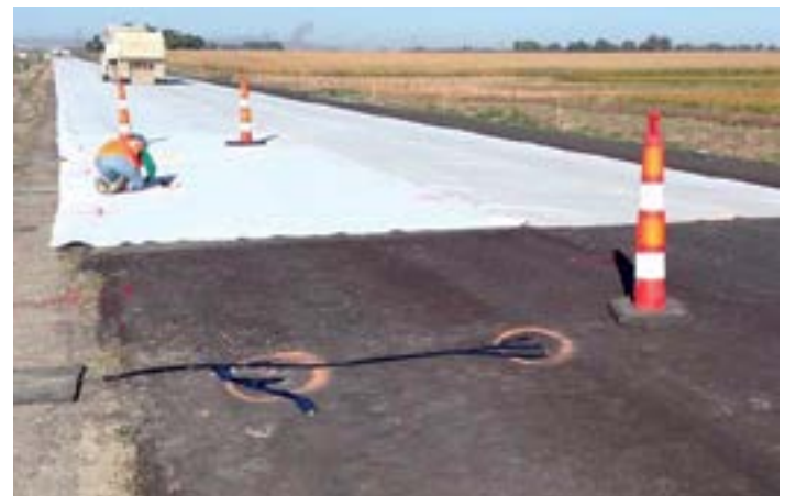
Figure 93. Light-colored geotextile fabric used as a separation layer for an unbonded overlay
