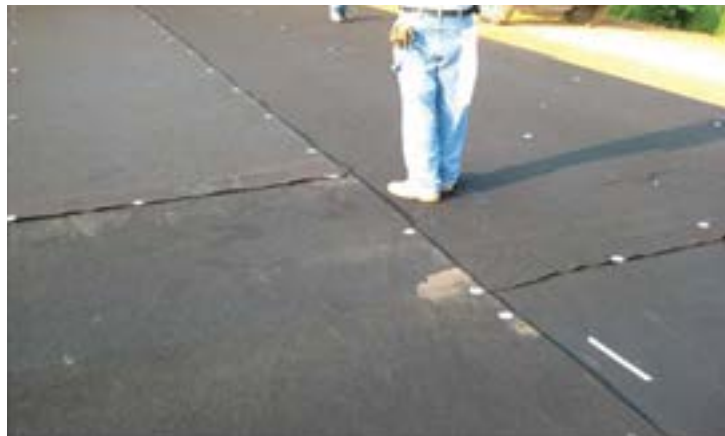
Figure 110. Overlap of nonwoven geotextile material section
