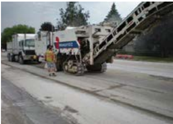
Figure 3. Milling concrete (left) and milled surface (right)
