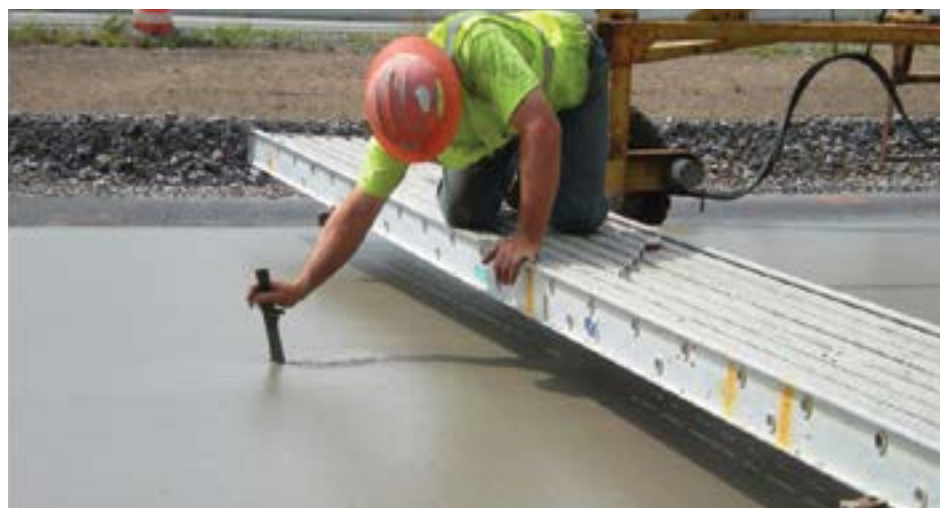
Figure 115. Manually verifying dowel placement
