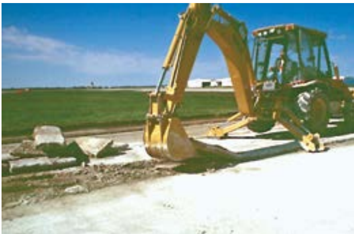
Figure 116. Removing overlay panels (source: Randell Riley, Illinois chapter, ACPA)
