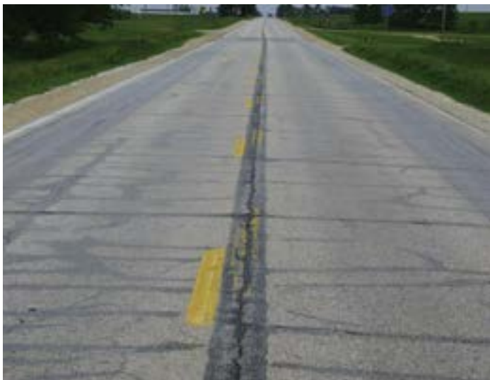
Figure 24. Existing composite pavement (source: James Cable, Iowa State University)
