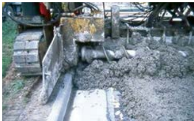
Figure 61. Concrete curb overlay (source: Jim Amundsen, Grace Construction Products)
