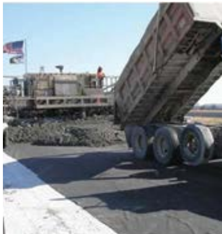
Figure 112. Paving on top of nonwoven geotextile materials
