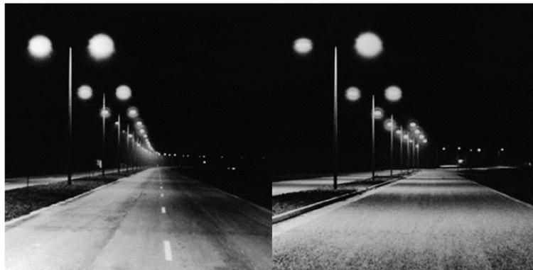
(a) (b) Figure 2. Specular vs. Diffused Pavement (Source: Van Bommel and De Boer 1980)
