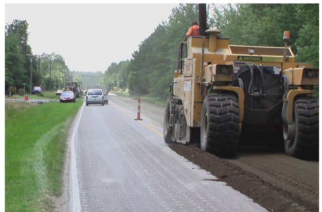
Figure 6.13. Pulverization of existing asphalt roadway
