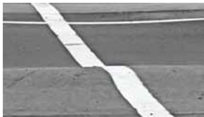
Figure 3.14. High-severity rutting
