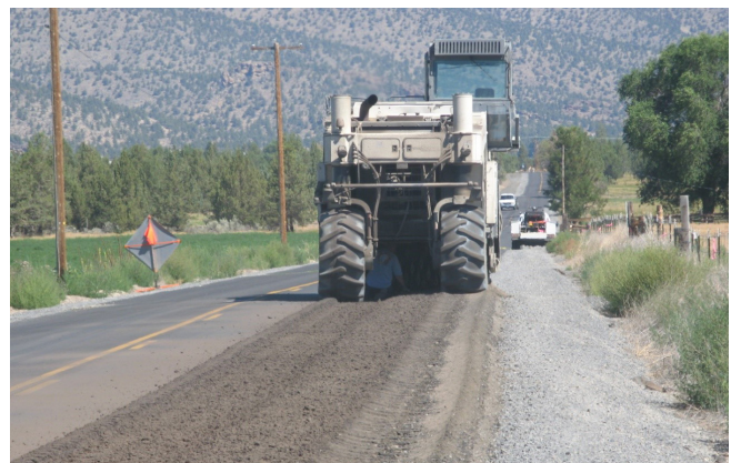
Figure 1.1. Road reclaimer performing FDR of an asphalt roadway
