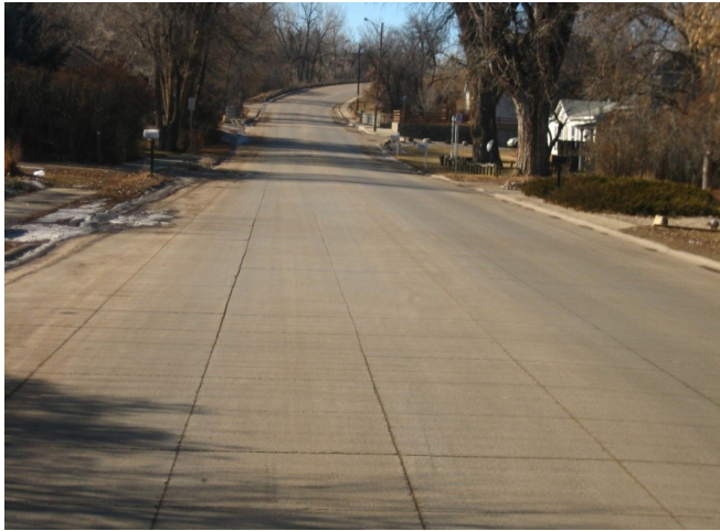
Figure 4.14. Bonded concrete overlay of FDR layer
