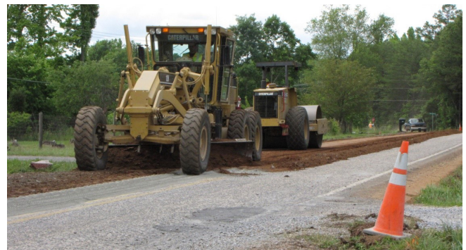
Figure 6.15. Grading of pulverized FDR mix
