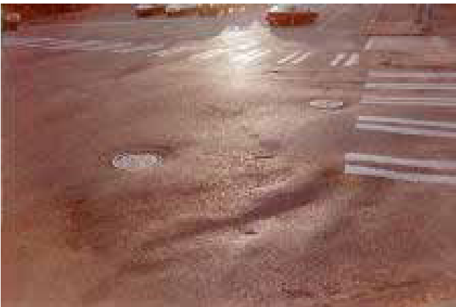
Figure 3.16. High-severity shoving
