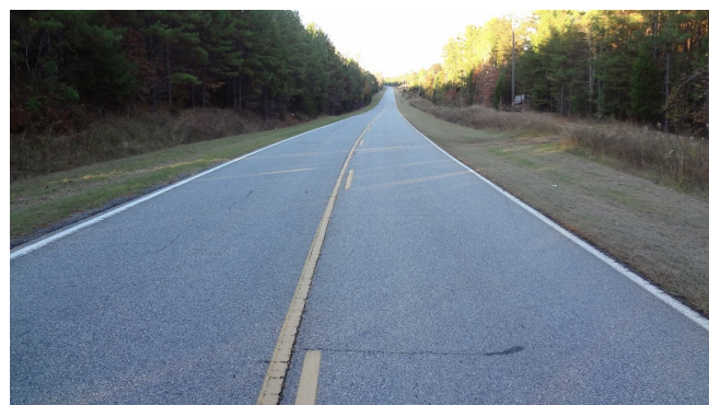
Figure 8.1. South Carolina state highway 97 (SC 97) is an FDR with cement project with excellent performance after 20 years of service
