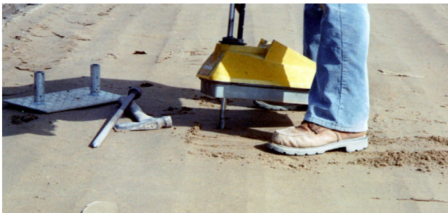
Figure 7.6. Density of compacted FDR being determined by a nuclear gauge in direct transmission mode
