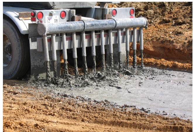
Figure 1.10. Application of cement slurry to pulverized mix
