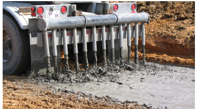
Figure 6.6. Cement slurry application
