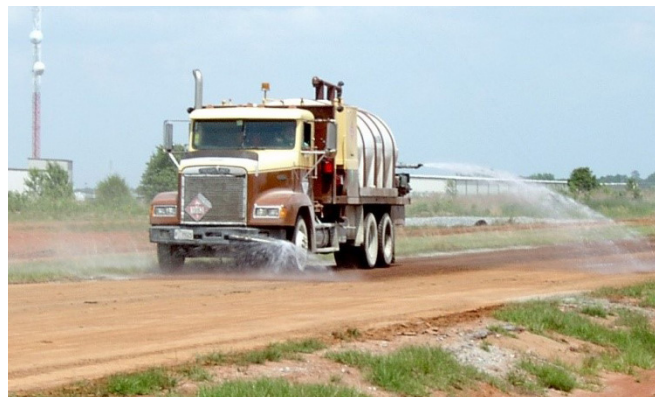
Figure 2.8. Water application on a compacted FDR base during the curing period
