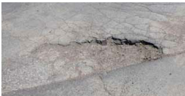
Figure 3.12. High-severity pothole
