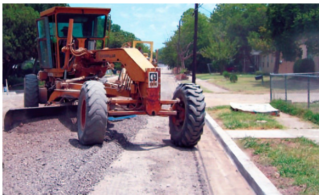
Figure 3.3. Aggregate being added to a roadway for minor alignment adjustments
