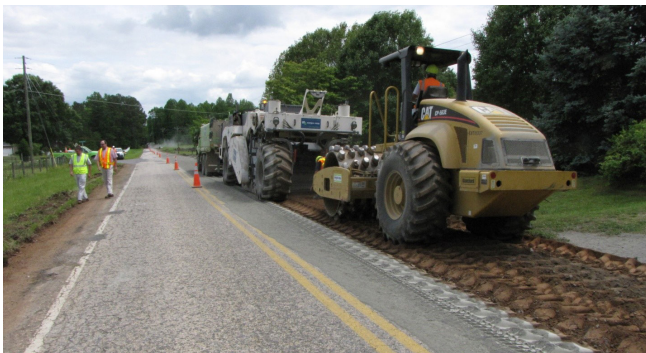
Figure 6.9. Tamping-foot roller behind reclaimer
