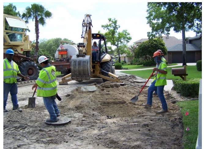
Figure 3.5. Existing utilities should be lowered before the pulverization process
