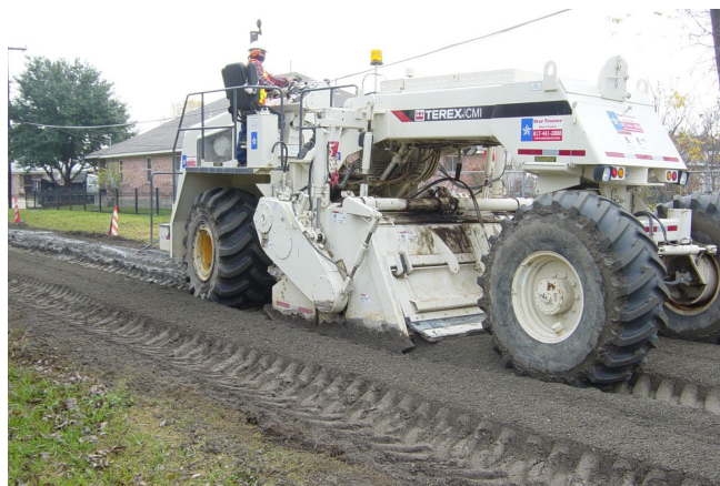
Figure 6.17. Cement slurry mixing operations
