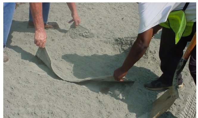
Figure 7.2. Cement application rate verification
