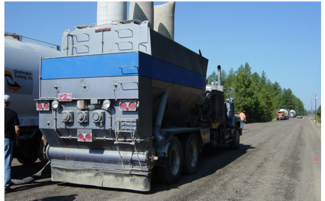
Figure 6.5. Self-contained vacuum system on a bulk cement spreader
