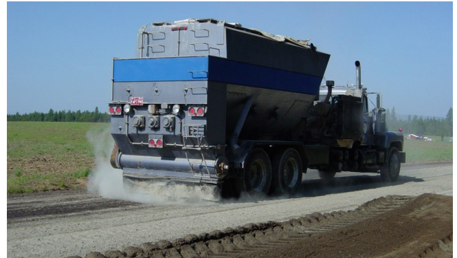
Figure 6.4. Dry powder cement being placed using a bulk spreader
