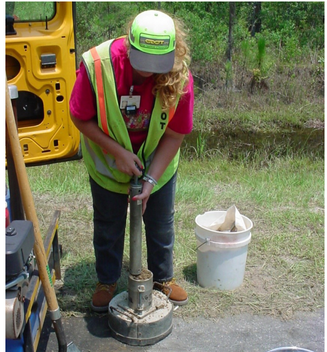
Figure 7.7. Proctor test during construction
