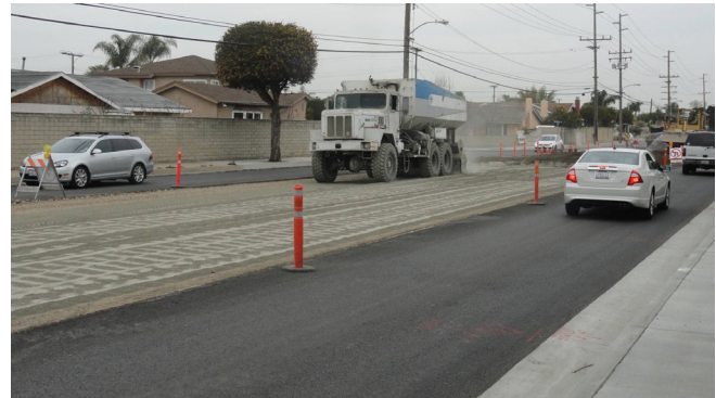
Figure 1.9. Application of dry cement powder to pulverized mix
