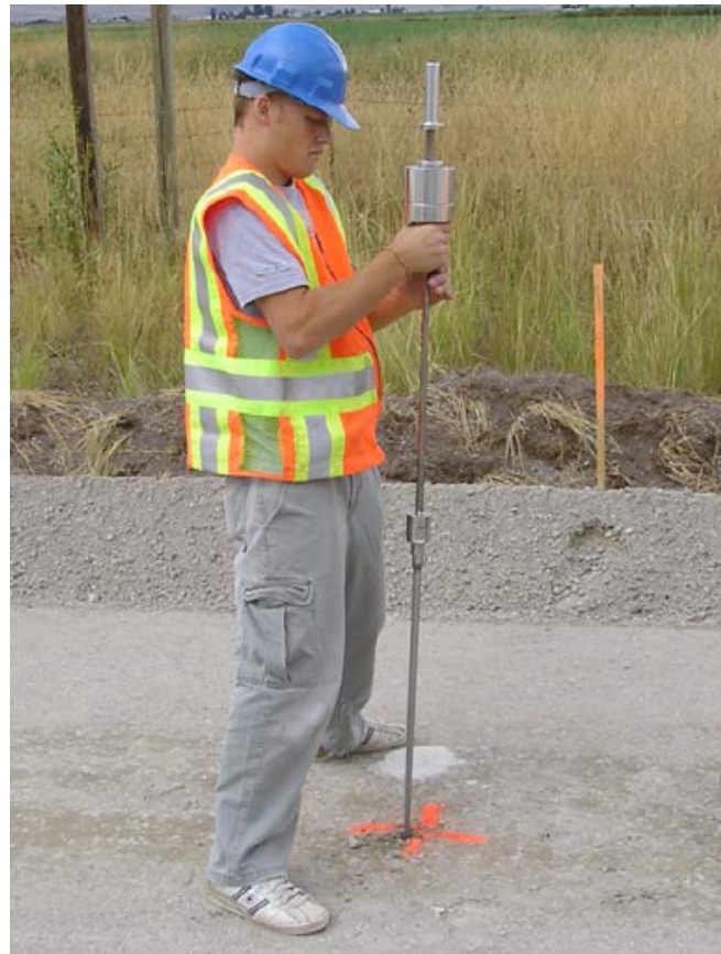
Figure 5.5. Dynamic cone penetrometer test
