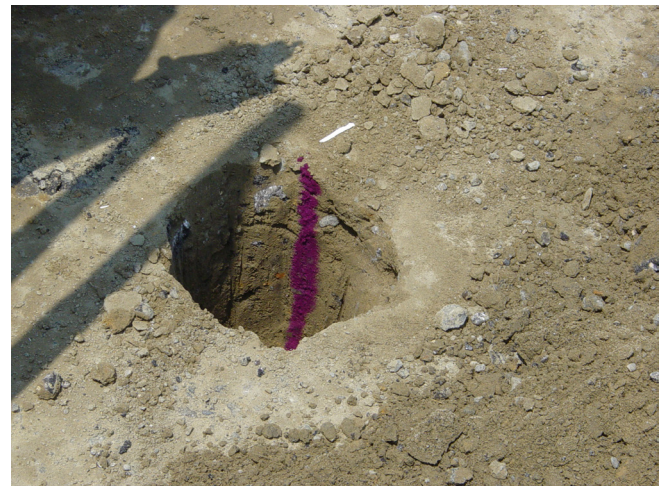
Figure 7.5. Checking depth of cement stabilization with phenolphthalein
