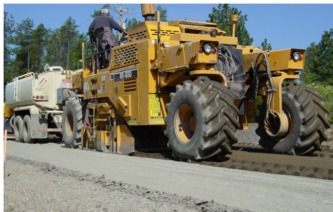
Figure 6.16. Mixing the pulverized material, dry cement, and water
