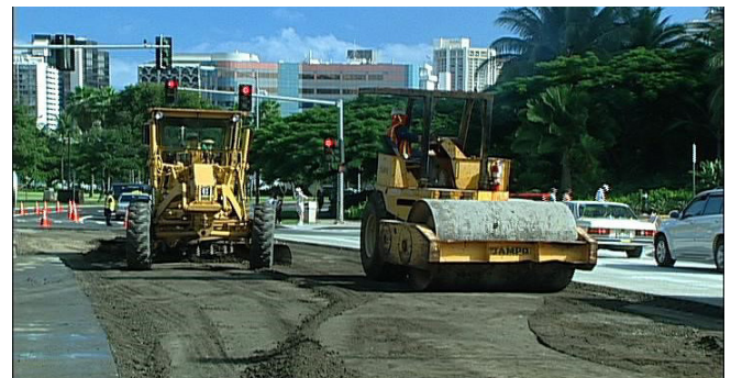
Figure 6.18. Compaction and final grading operations
