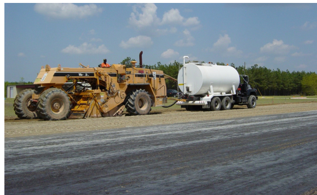
Figure 1.17. FDR construction of airport runway
