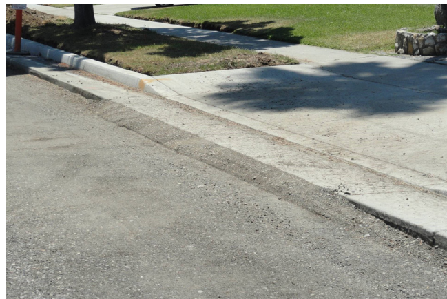
Figure 1.16. This compacted FDR base was opened to light residential traffic before application of surface course
