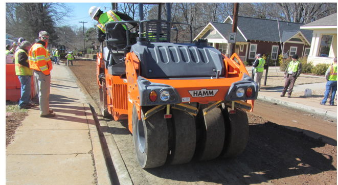
Figure 6.10. Finish rolling using pneumatic tire roller
