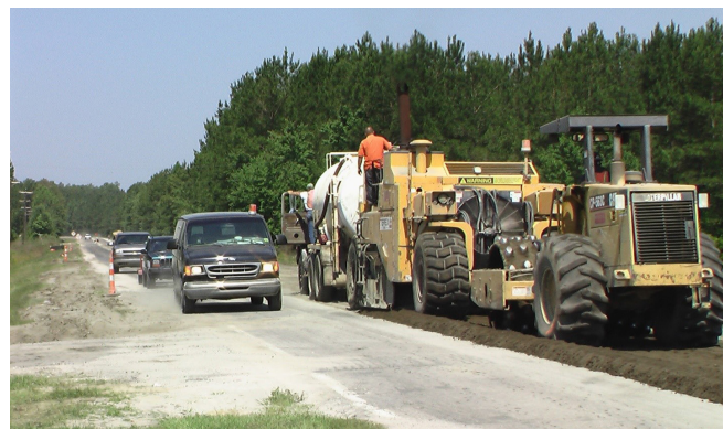
Figure 6.20. Full-depth reclamation while maintaining traffic
