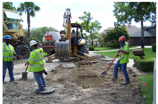
Figure 1.7. Utilities like this manhole may need to be lowered beneath the proposed FDR depth before construction
