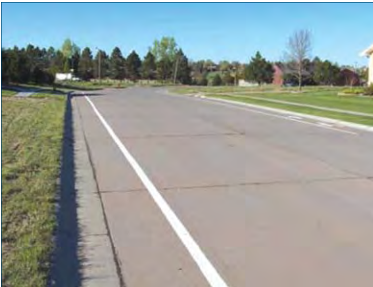
Figure 2-5. RCC pavement used for a local street
