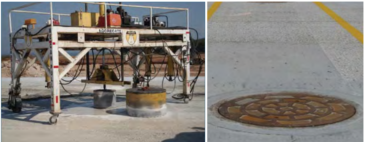
Figure 7-15. Coring (left) and isolation joint (right) around a manhole
