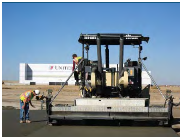
Figure 2-3. RCC paving operation at an airport
