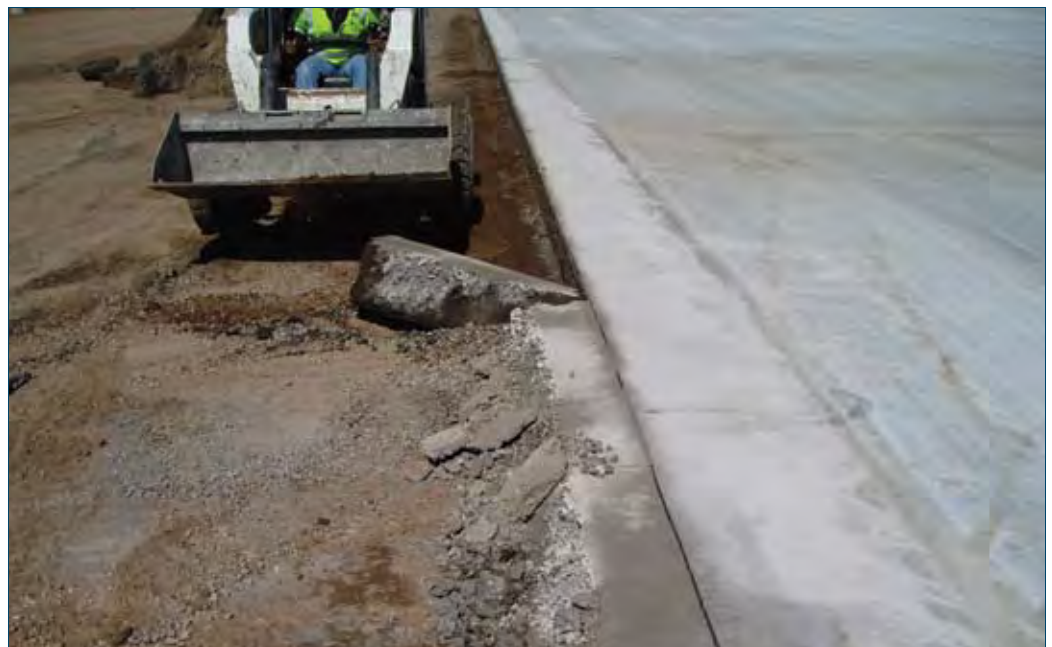
Figure 7-7. Finished longitudinal construction cold joint
