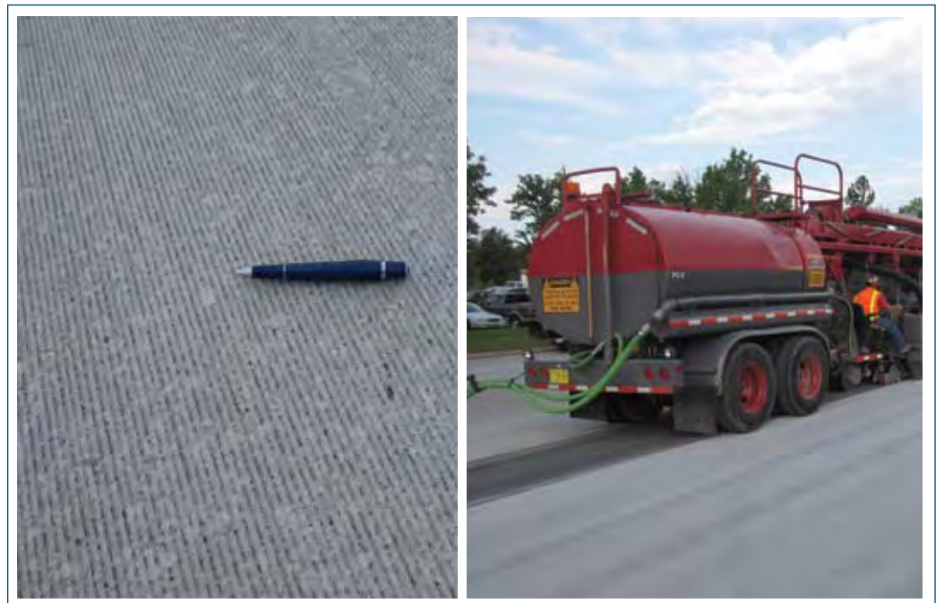
Figure 1-9. Diamond grinding of RCC provides for a smooth and quiet surface
