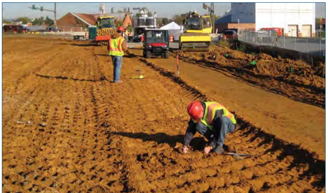
Figure 7-1. Preparation of subgrade
