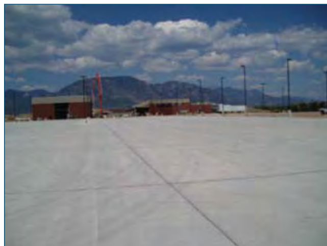
Figure 7-12. Sawn transverse and longitudinal joints
