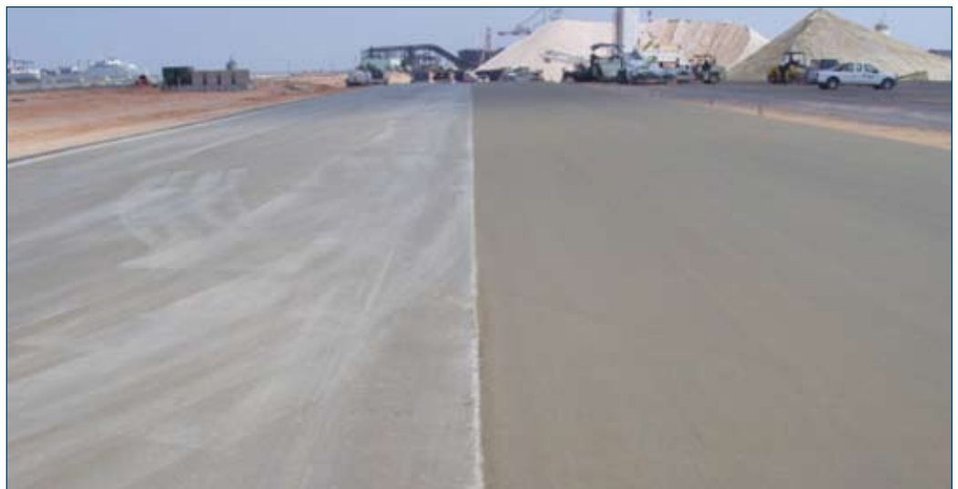
Figure 7-14. Longitudinal construction joint
