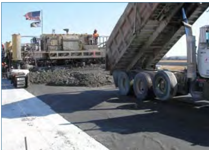
Figure 2-7. Concrete paving with geotextile fabric layer
