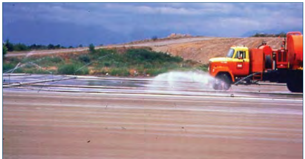
Figure 7-17. Moisture curing using sprinklers and fog spraying
