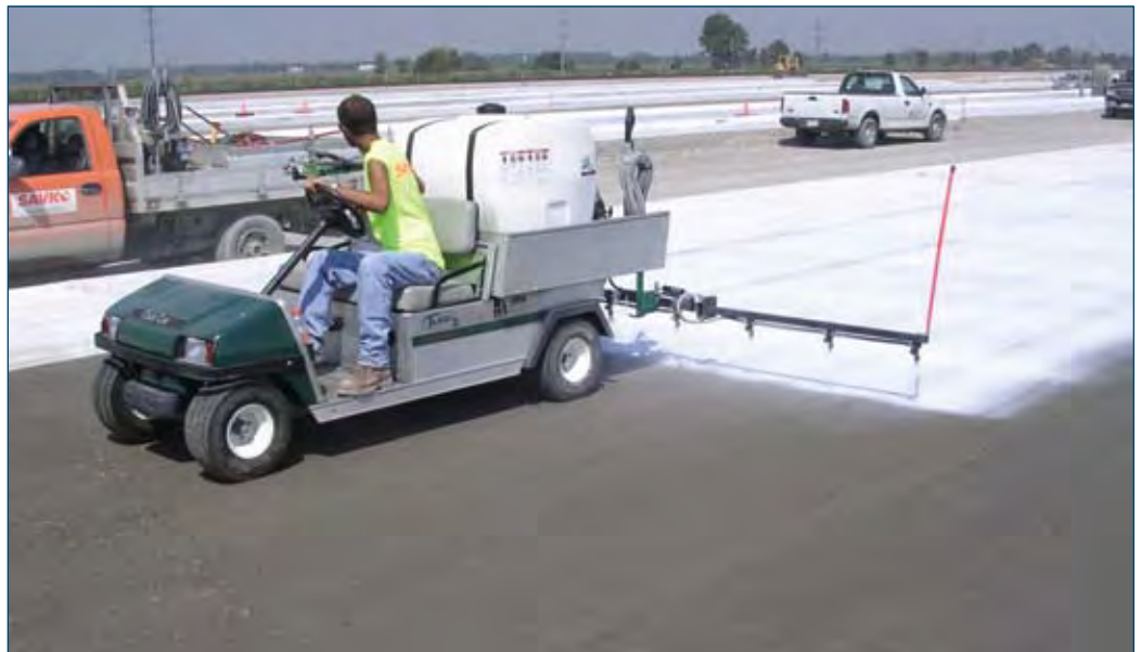
Figure 7-16. Application of curing compound
