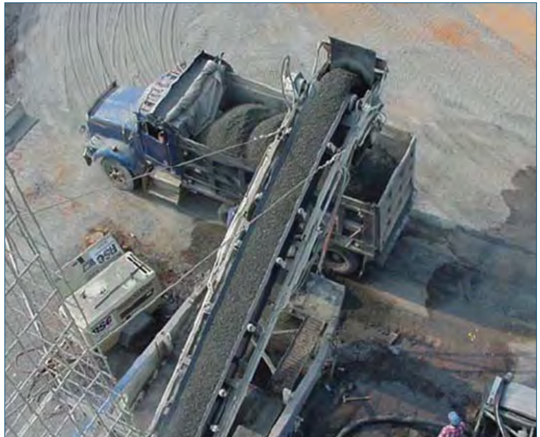
Figure 7-2. RCC uniformly loaded into dump truck (California and PCA)
