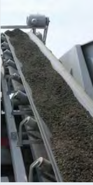
Conveying RCC from mixer to be loaded into dump truck
