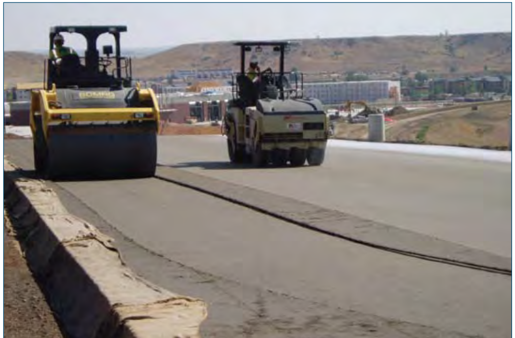
Figure 7-5. Side-by-side view of steel drum and rubber-tired rollers (Edwards)
