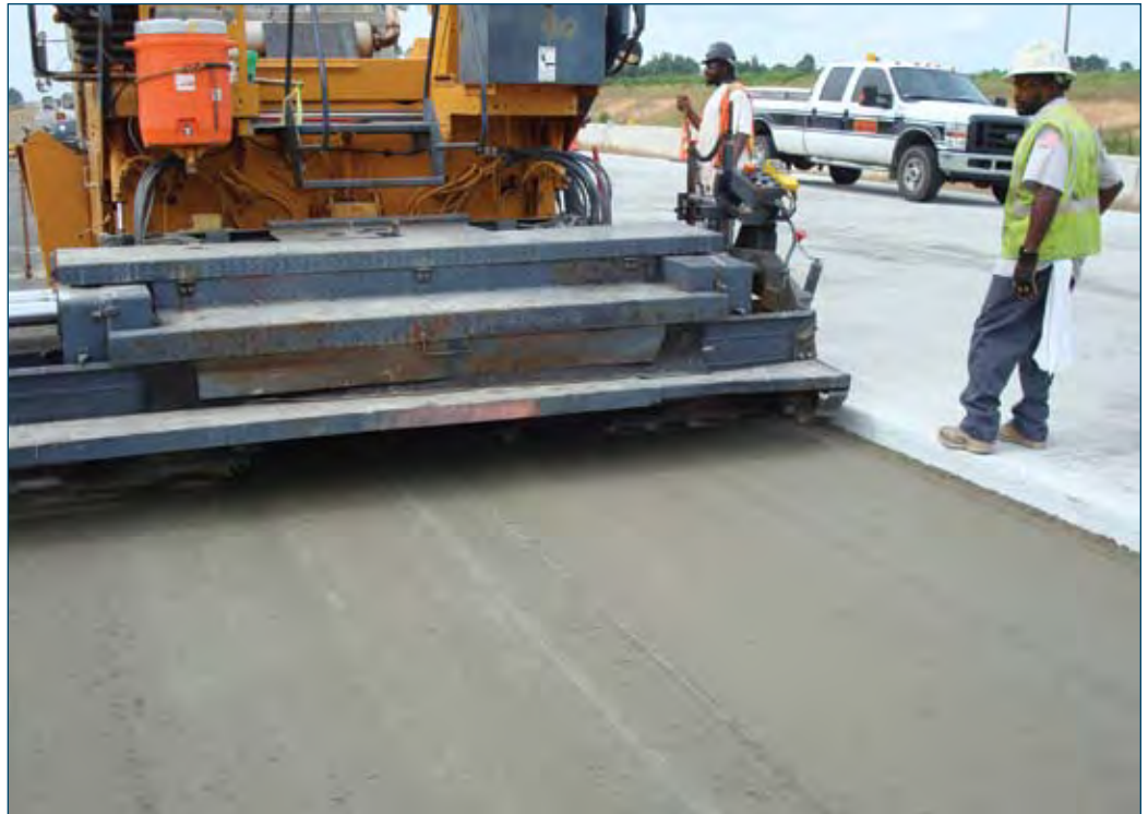
Figure 7-4. Close-up view of paver
