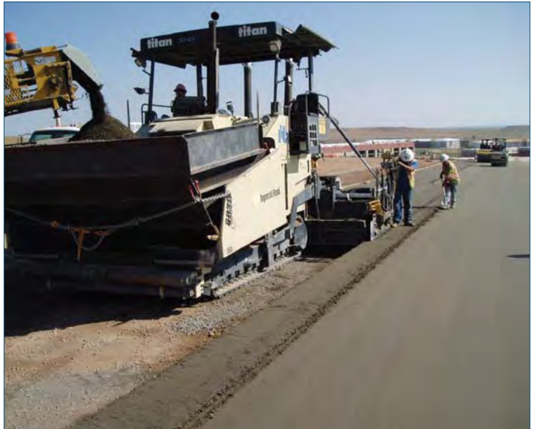
Figure 7-6. Fresh longitudinal joint
