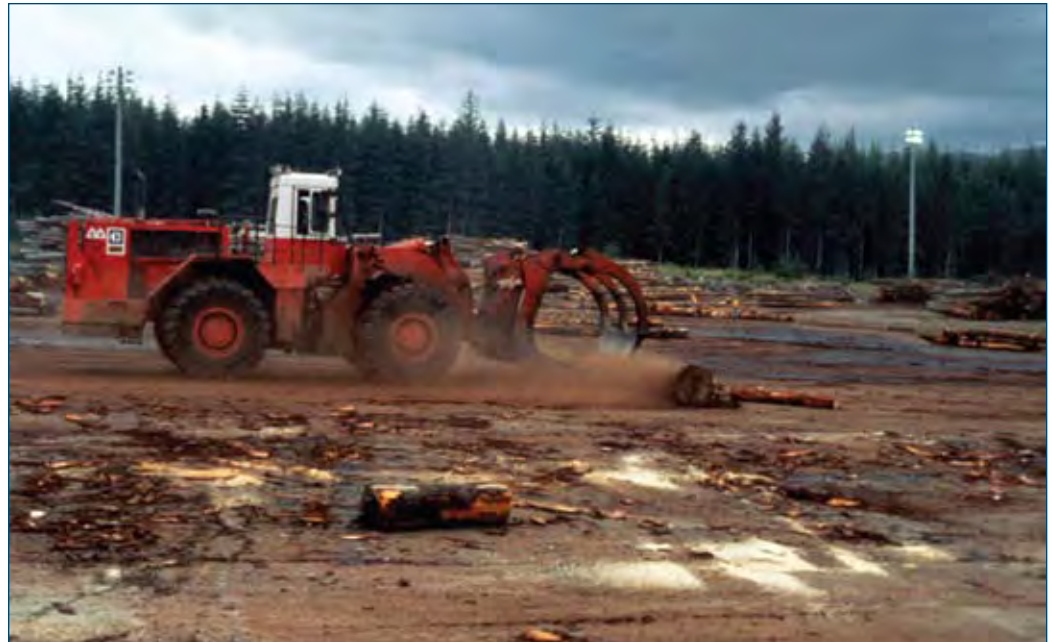
Figure 2-8. RCC pavement constructed at a log handling facility
