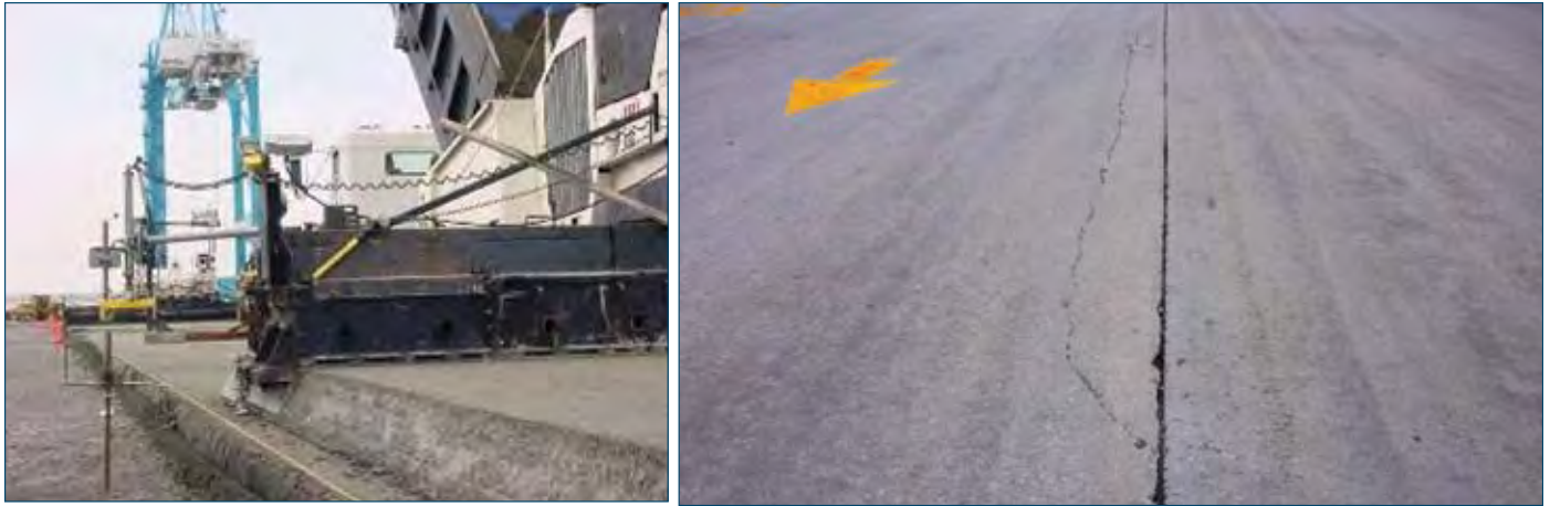
Figure 7-8. Paving shoe (left) used on the second lift, and longitudinal crack from first lift joint reflecting through adjacent second lane (right)
