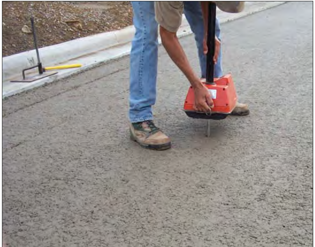
Figure 7-3. Checking density using a single-probe nuclear gauge
