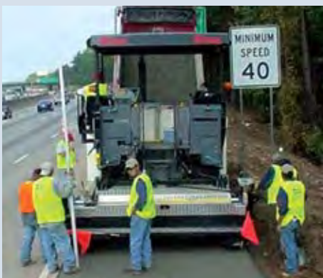
Interstate highway shoulder, Atlanta, GA
