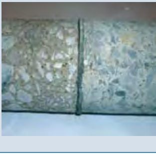
Pavement core showing multi-layer system with geotextile fabric layer
