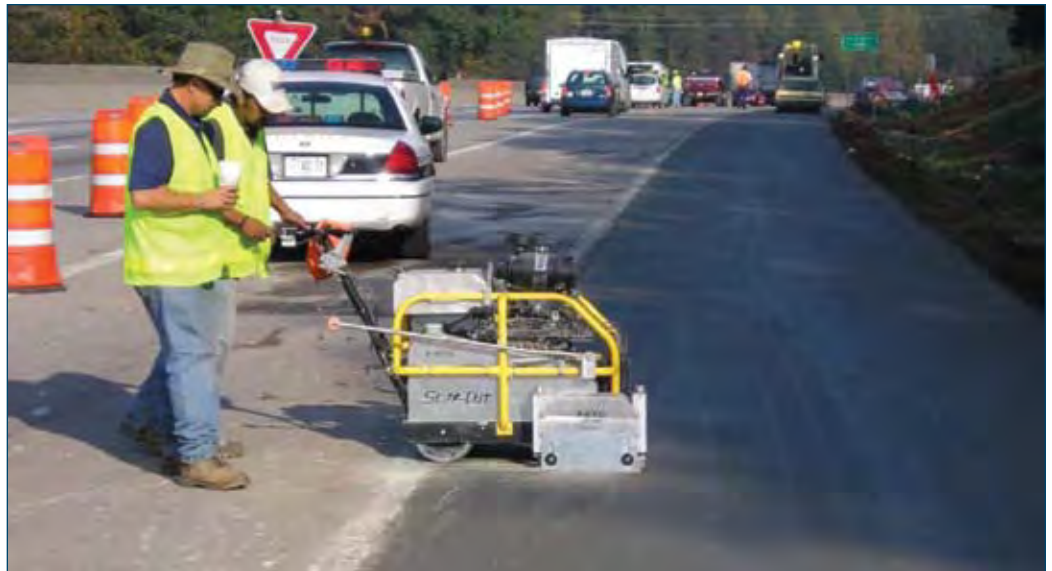
Figure 7-13. Shoulder transverse sawed joint
