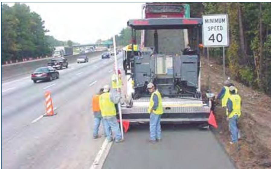
Figure 2-6. RCC used to reconstruct shoulders on I-285 near Atlanta, GA
