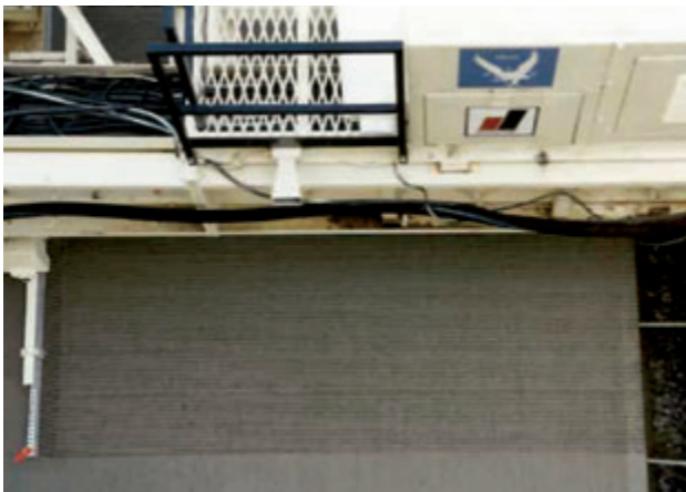
Figure 6.5. Transverse tining (uniform spacing) of a plastic concrete pavement surface. 110
