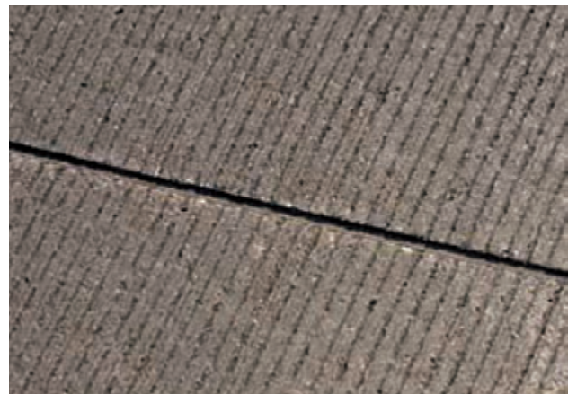
Figure 6.8. Concrete pavement surface textured with longitudinal tining.
