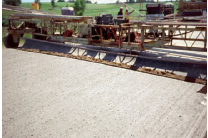
Figure 6.3. Photos of aggregate weighting on Astroturf drag (photos provided courtesy of Mr. Doug Schwartz, Minnesota DOT).
