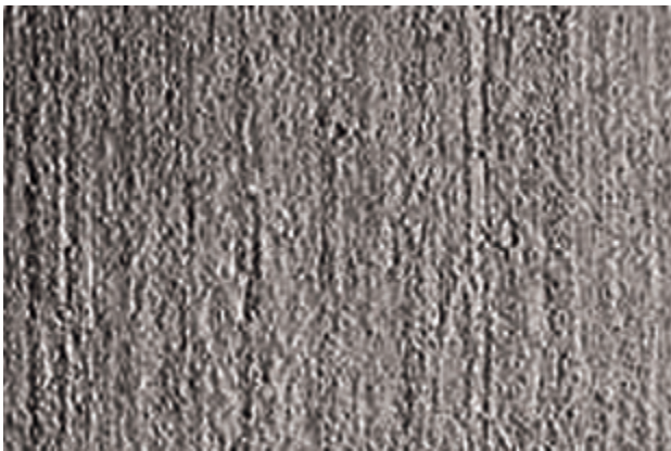
Figure 6.1. Photograph of a typical concrete surface created using burlap drag.
