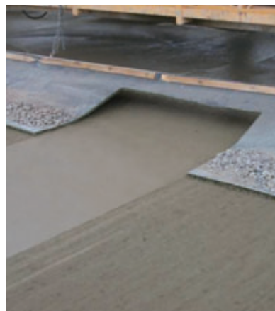
Figure 6.3. Photos of aggregate weighting on Astroturf drag (photos provided courtesy of Mr. Doug Schwartz, Minnesota DOT).
