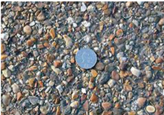
Figure 6.9. Close-up photograph of an exposed aggregate concrete pavement surface. 172
