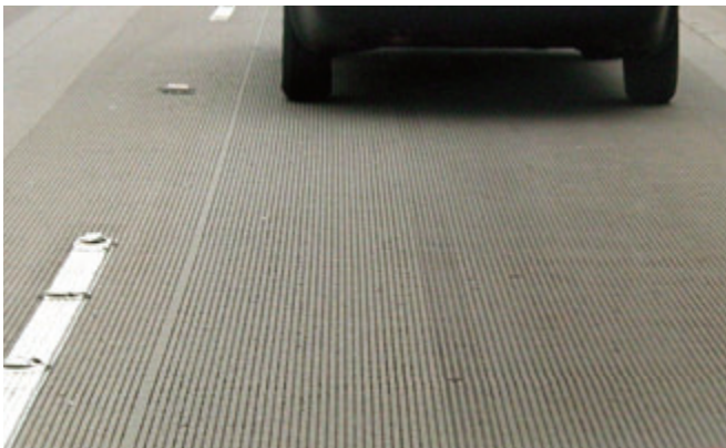
Figure 6.16. Photo of longitudinal grooving. Photo courtesy of Dr. Michael Darter, ARA Inc.
