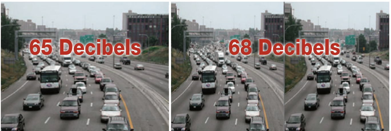
Figure 3.3 Doubling traffic flow (with constant composition) increases sound by about 3 dB.
