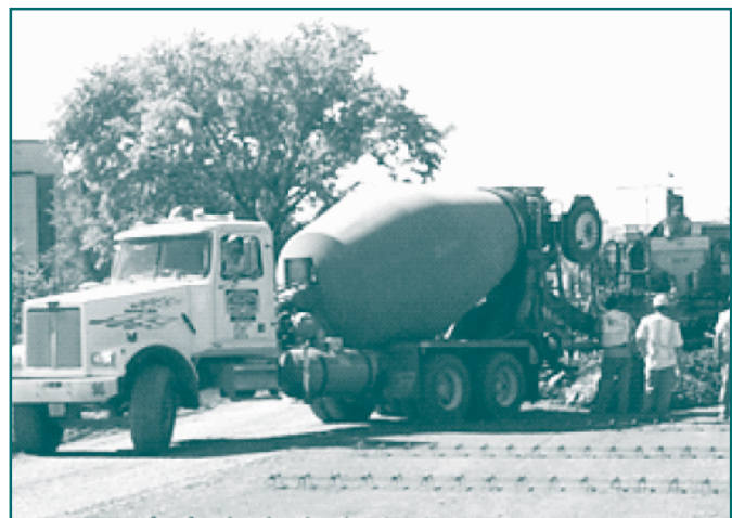
Figure 1b. Dowel baskets positioned ahead of paver
